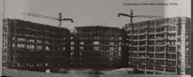
Construction of New Main Building (1970s)
